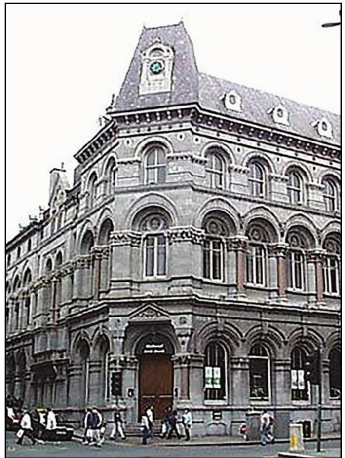
The former Danske Bank branch in College Green, which is due to open shortly as a new outlet for the H&M fashion chain.
